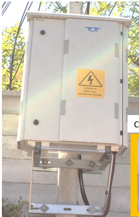
19" Aluminum Outdoor Cabinet 840 Fiber on pole
