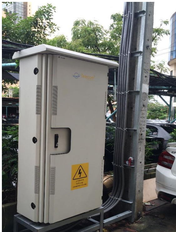
19" Aluminum Outdoor Cabinet 1200 Fibers for floor
