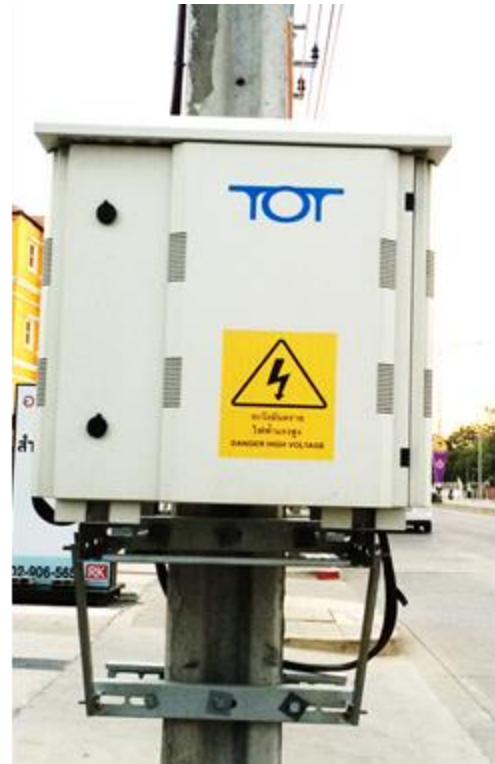
19" Aluminum Outdoor Cabinet 288 - 540 Fibers on pole
